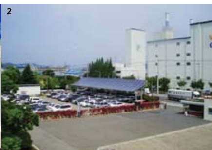
1. Conclusion of cooperation agreement against climate change with Korea Environment Corporation 2. Solar panel installed in Gumi 1 site's parking lot
